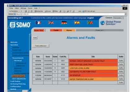
Alarms and faults
